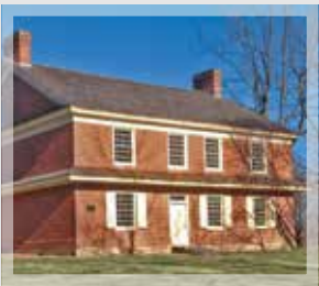
Primitive Hall (830 N. Chatham Rd. West Grove)
